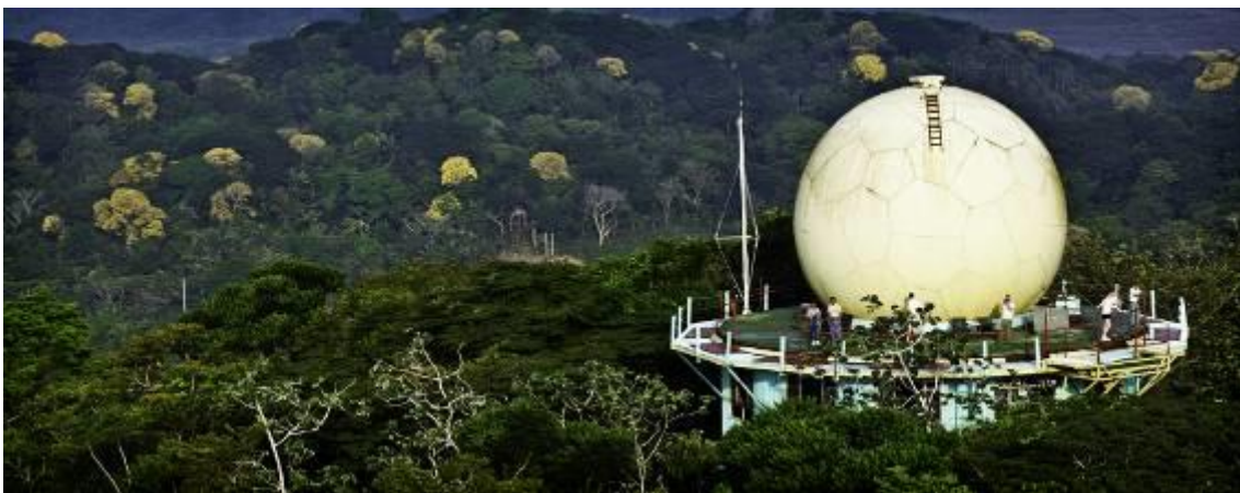
Canopy Tower (photo courtesy Canopy Family)
